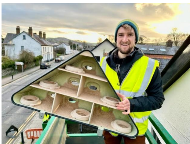
Project volunteer Ben Porter with a 6 chambered 'Impeckable' design apex Swift box which was installed on the Machynlleth Co-op store.
